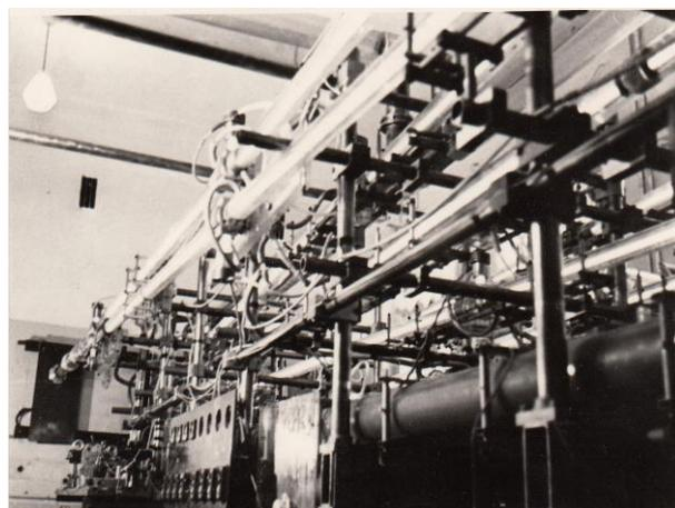
**Figure 7.** "Zig-Zag"- CO<sub>2</sub>-laser created by A.I. Barchukov FIAN 1970.
